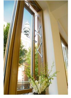
All open with a two handed operation using handles mounted on either side of the oak vent.
